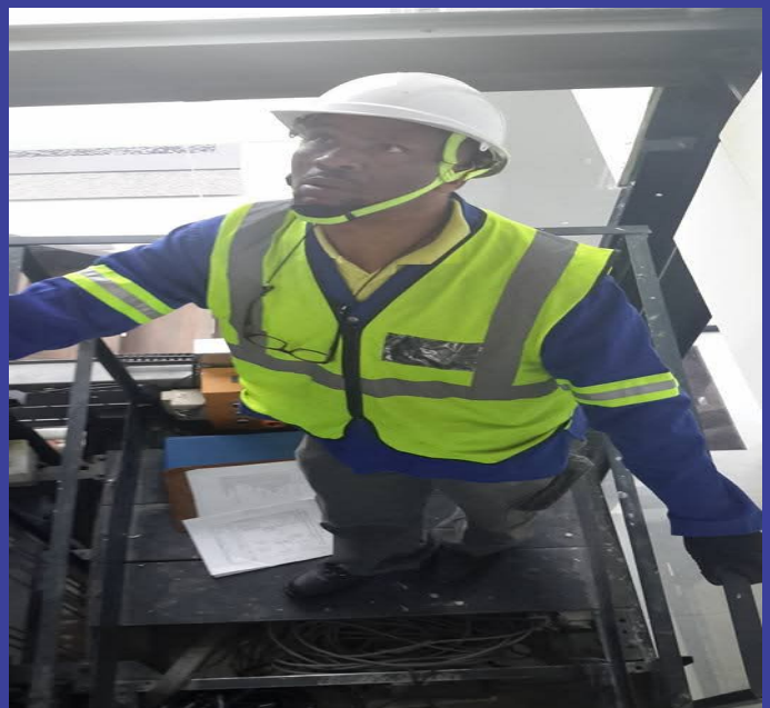
CONDUCTING TOP OF CAR INSPECTION
